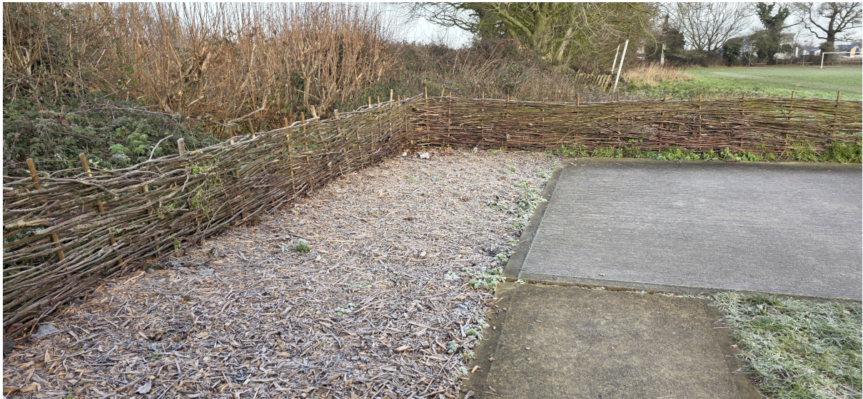
Figure 13: Wattle fence made from hedgerow branches beside the concrete pad
